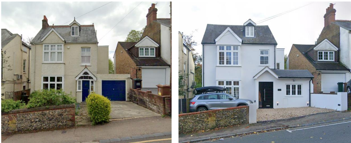
The application dwelling prior to any works in 2024 (left), and following completion of works in 2025 (right)
